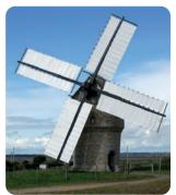
Our mill is what we call a "petit-pied" mill: its typical architecture has a base that is narrower than its head.
